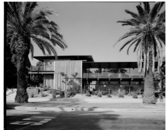
Photo: Classroom Building Sequoyah School Photo Source: Library of Congress
